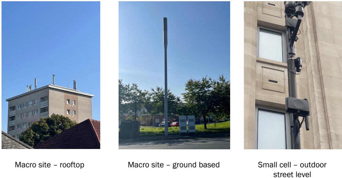
Figure 3.4: Examples of macro site vs. small cell [Source: Analysys Mason, 2023]
