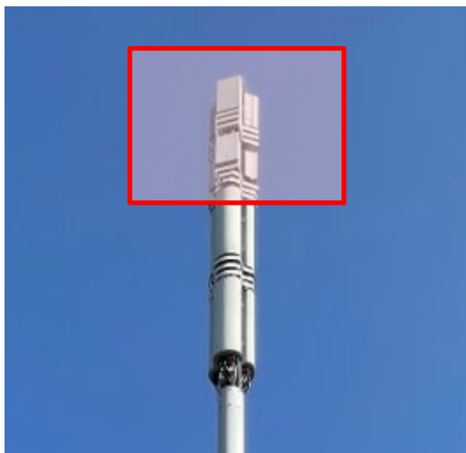
Additional antennas, increasing the tower height
