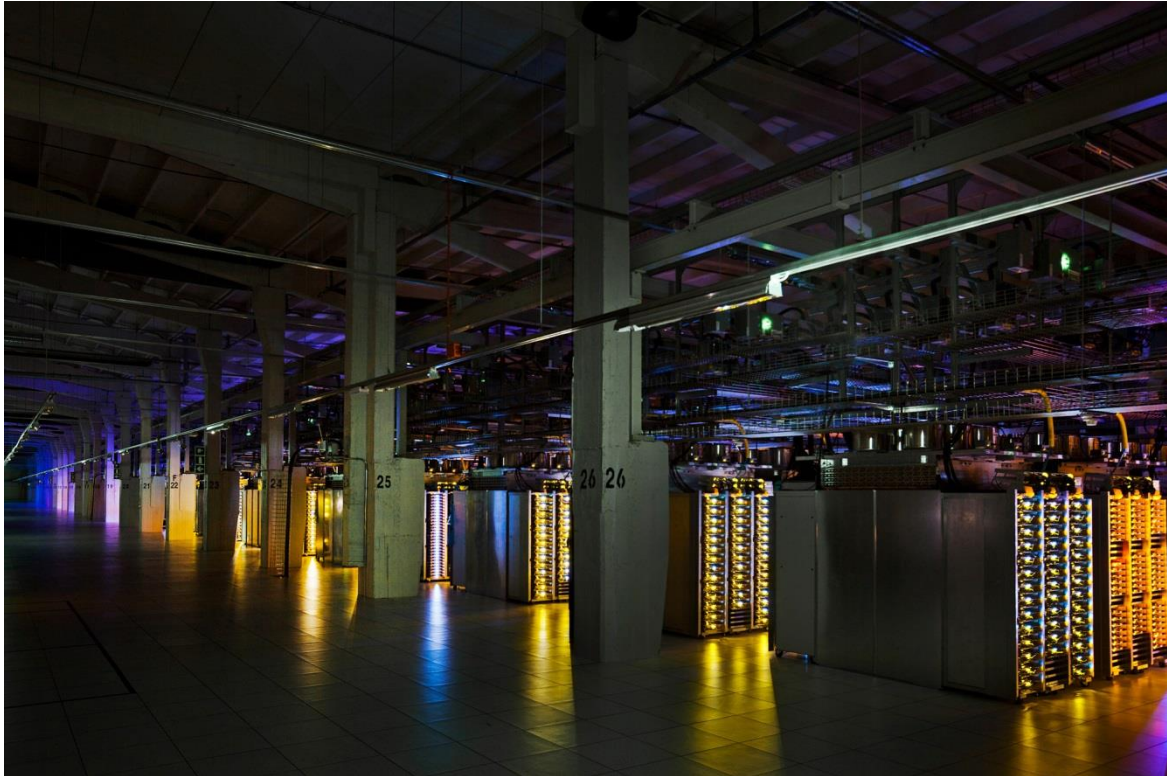
Figure 4.2: Interior of Google's Hamina data centre, showing racks for the housing of servers and storage devices, and other systems [Source: Google, 2014]
