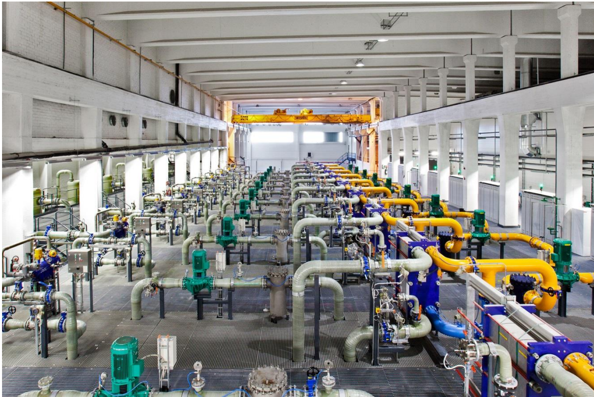
Figure 4.5: Cooling system at Google's Hamina data centre [Source: Google, 2014]
